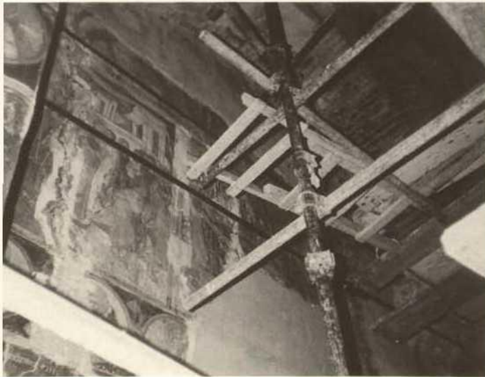
Petkovic Monastery, conservation work on mural painting
