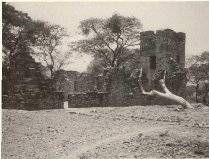
Niamkolo church ruin, built in 1896 – currently a national monument. The ruin suffered from vandalism by locals removing stones to repair their own houses.
