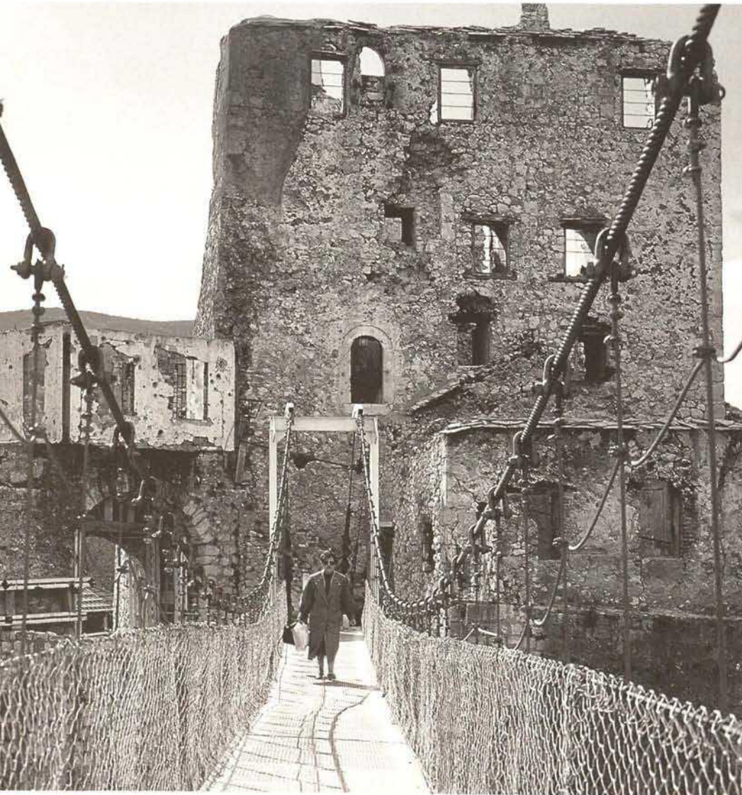
Temporary suspension bridge in Mostar (in the meantime replaced by a reconstruction of the old bridge)
