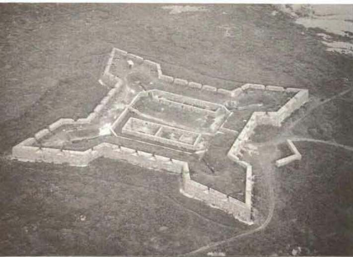
Bird's eye view of Fort Prince of Wales, fortress of Vauban type (1731–71), Churchill, Manitoba
