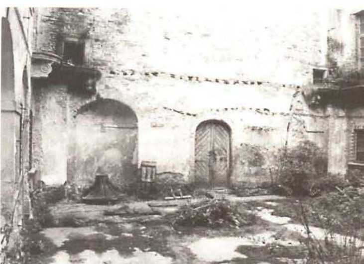
Bečváry (Kolín district): view into the courtyard
