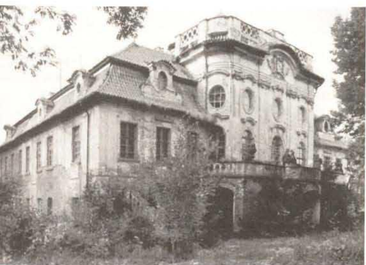
Bečváry (Kolín district): main façade as seen from the park
