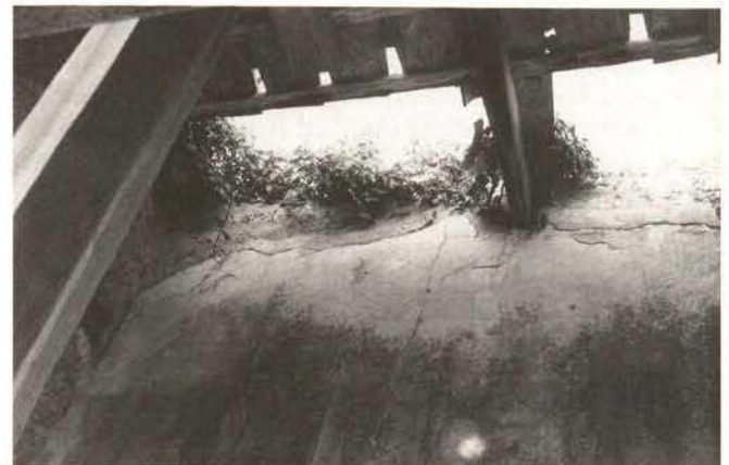
A gap in the protective roof. Ivy has come through and has already grown over the top of the wall.
