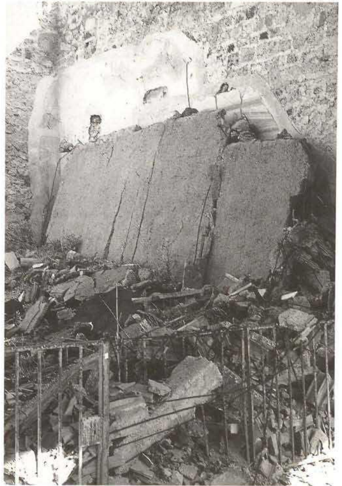
Collapsed parts of a reinforced ceiling of concrete and bricks, leaning against the wall painting behind, which itself is without any protection against bad weather (Casa Labyrinth).
