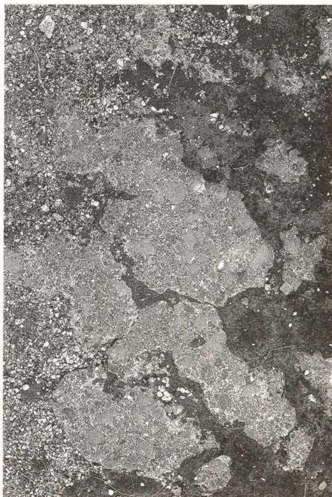
Remains of heavily damaged floors with inlaid brick fragments - the original floors in Pompeii are not only damaged by weathering but are often trodden on by the tourists (Casa dei Postumii).
