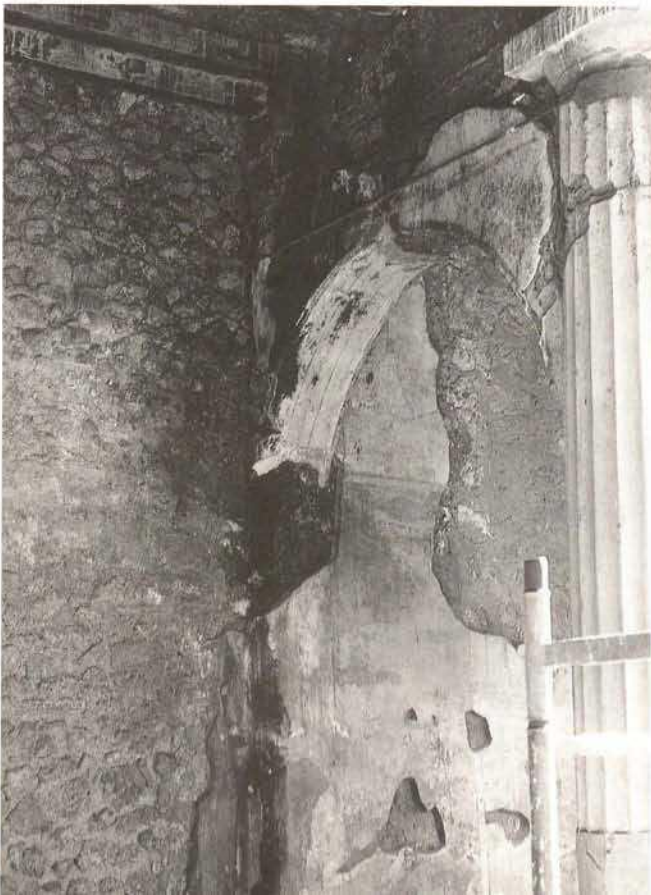
Decay of the modern ceiling construction (brick with iron reinforcements) above the original wall decoration which is already heavily damaged by pervading water (Casa Rebio Valente).
