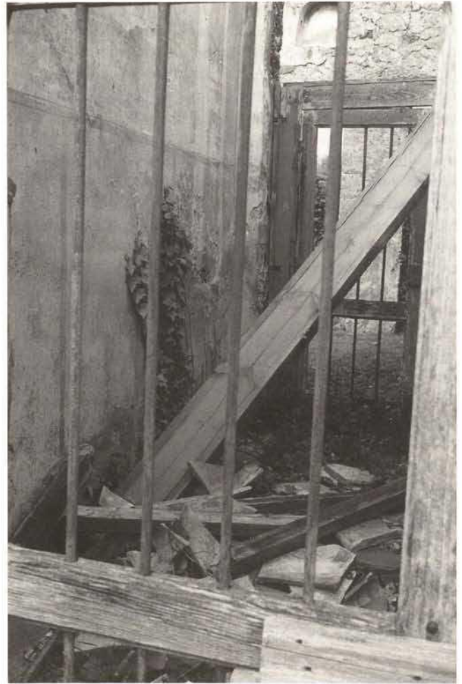
Condition of a decayed "taberna". The collapsed construction material is lying around and dilapidated. The "taberna" was excavated 90 years ago and was once decorated with well-preserved wall paintings.
