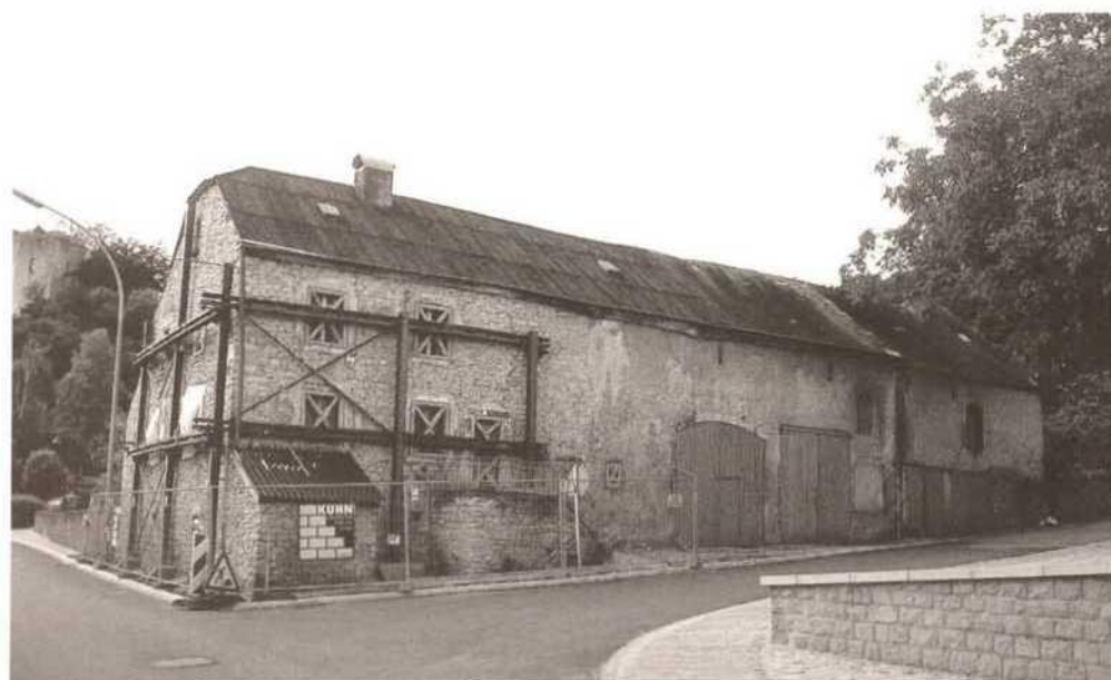
Septfontaines, rescue of a house threatened by road construction
