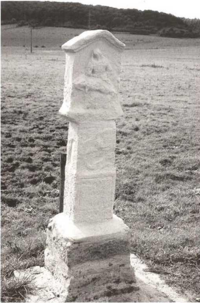
Steinsel, wayside cross after restoration
