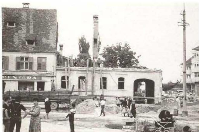
Sighișoara (Schäßburg), demolition of the historic mill district during Ceaușescu's time (1986)
