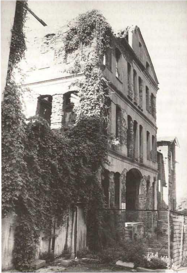
House at Süleymaniye. Fires caused serious losses to the historic fabric of Istanbul which consisted mainly of timber houses. Many of the houses in Süleymaniye are made of timber; occasionally they burn and are replaced by reinforced concrete copies. This house is built of brick but it had timber floors and roof. It suffered from a fire about ten years ago and due to lack of funds stands as a ruin.
