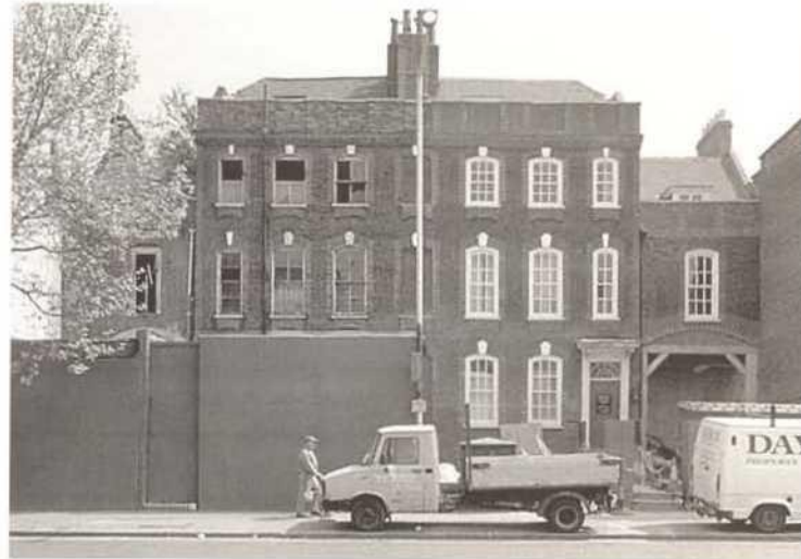
810 Tottenham High Road (c1715), Haringey, London. A symmetrical pair of grade II* listed houses; the one on the right has been repaired while the other remains at risk.
