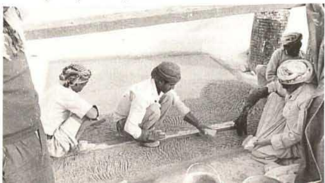
Pounding of a quadath layer
