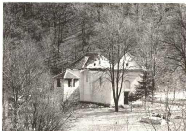
The village of Ba, church damaged by earthquake
