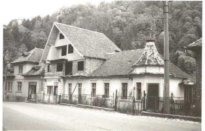
Romania, Bran village – the results of modernisation (1998)
