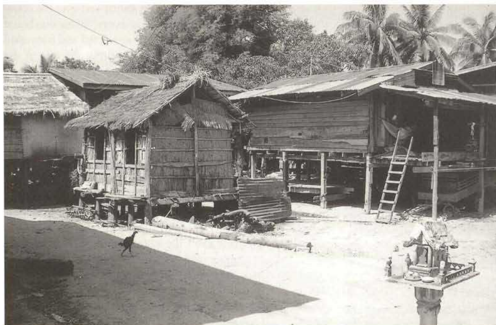
Thailand, village in the Sukhothai area, traditional farmstead, the roofing has been replaced by corrugated iron (1997)
