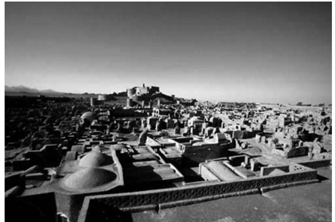
Fig. 1 The Arg and the other historic buildings of the city as symbols of Iranian art and tradition
