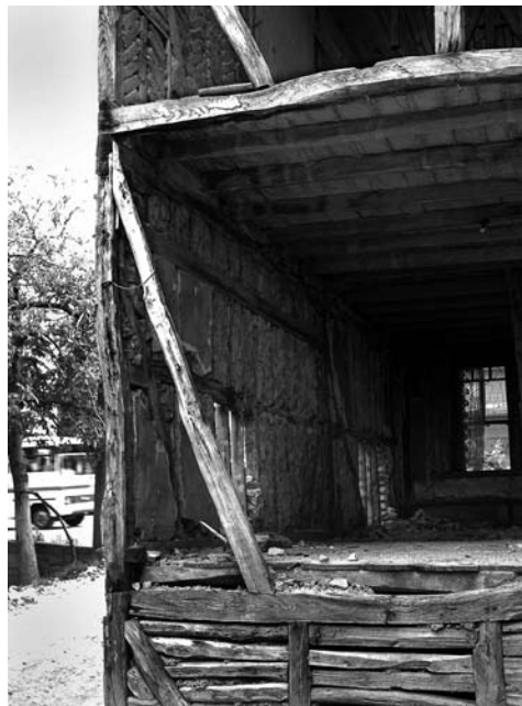
Figs. 14 and 15 Partially demolished house in Gölcük at the time of the earthquake showing the single brick wythe thickness of typical humuş wall. Fig. 14 shows the exterior and fig. 15 the interior face of the same wall. Despite its condition, the earthquake had little affect on it. 2003 (photographs © Randolph Langenbach)
