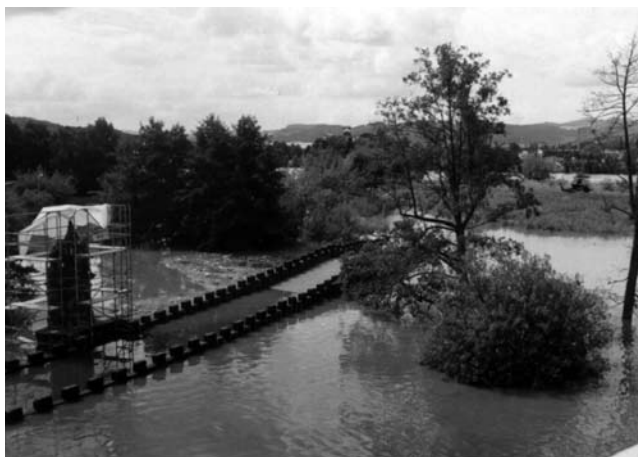
Fig. 9 Děčín, stone bridge in the late medieval Gothic style with a sculptural group of St. Vitus, St. John of Nepomuk and St. Wenceslas by the sculptor M. J. Brokof from 1714. One of the pillars was damaged by the flood and the bridge statics was affected.
