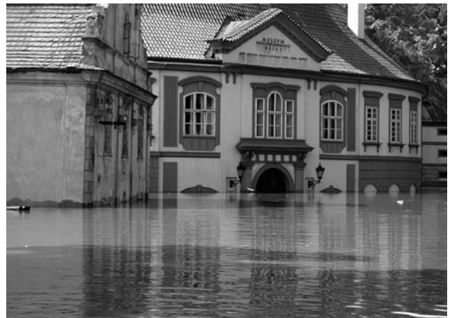
Fig. 6 Liběchov, historic country house and park, an important Baroque building by the excellent Czech architect F. M. Kaňka, built about 1730, with a park established in a formal style and decorated with numerous sculptures. The historic country house was flooded up to a height of 3.5 meters. Very valuable wall paintings by the well-known Czech painter Josef Navrátil are in critical condition. The valuable park was devastated and muddied.
