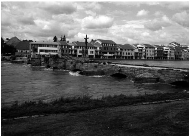
Fig. 5 Písek, the oldest medieval stone bridge in Bohemia from the period after 1250 with Baroque sculptural decorations. The bridge was completely under water, the breastwork walls made of granite square stones and one copy of the Baroque statues collapsed because of the flood.
