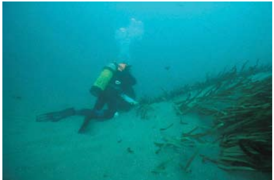
Figure 2: Build up of stabilised sand following placement of artificial sea grass matting
