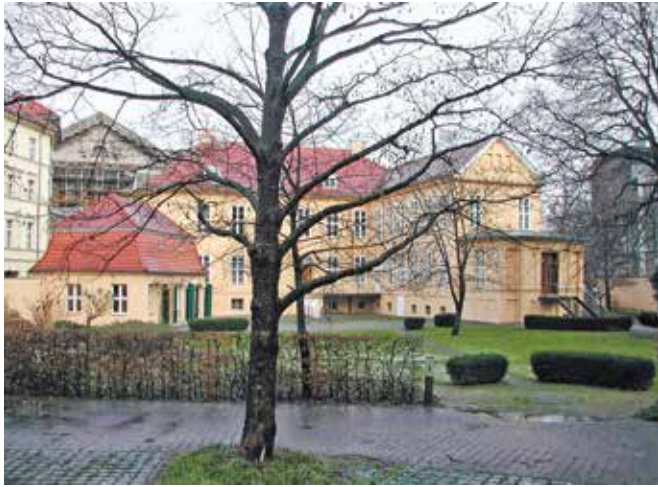
The rear front of the Magnus-Haus and the open space of the garden belonging to it
