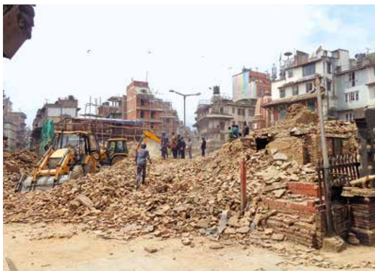
Collapsed Kastamandap, the oldest monument which gave Kathmandu its name (meaning wooden structure), regrettably being cleared using excavators
