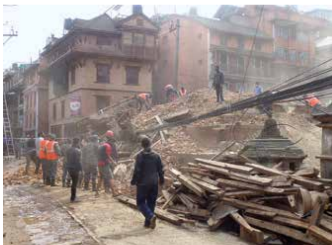
Community and armed forces helping to salvage from a collapsed temple in Patan
