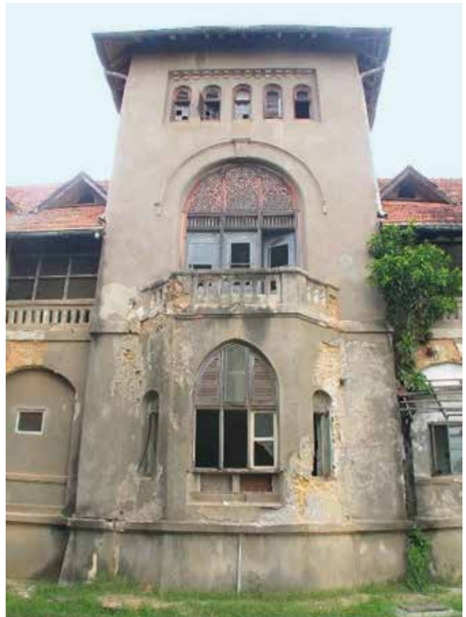
Oriel window at the rear side
