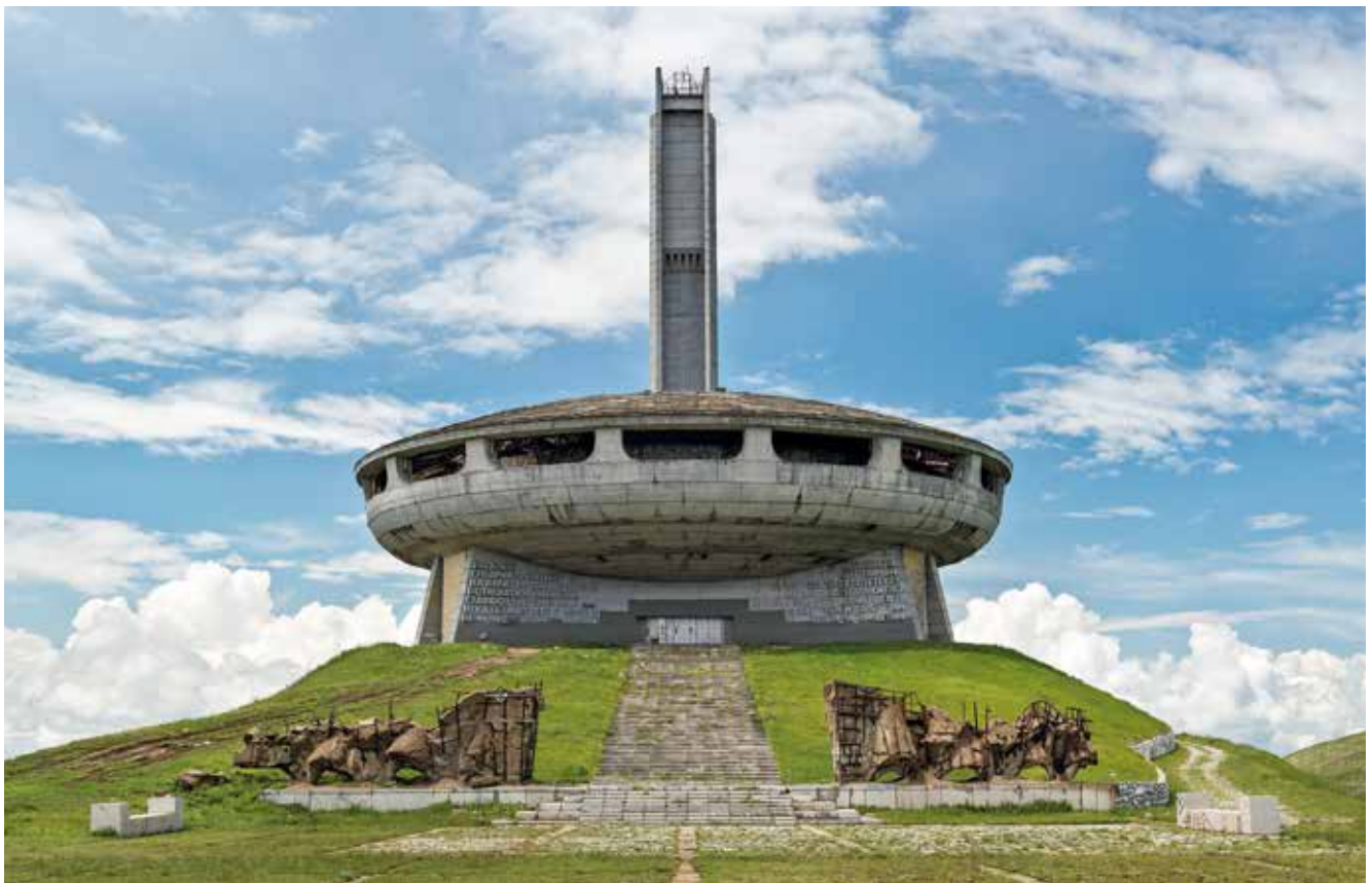
Fig. 1: View of the Buzludzha monument today (photo Les Johnstone)
