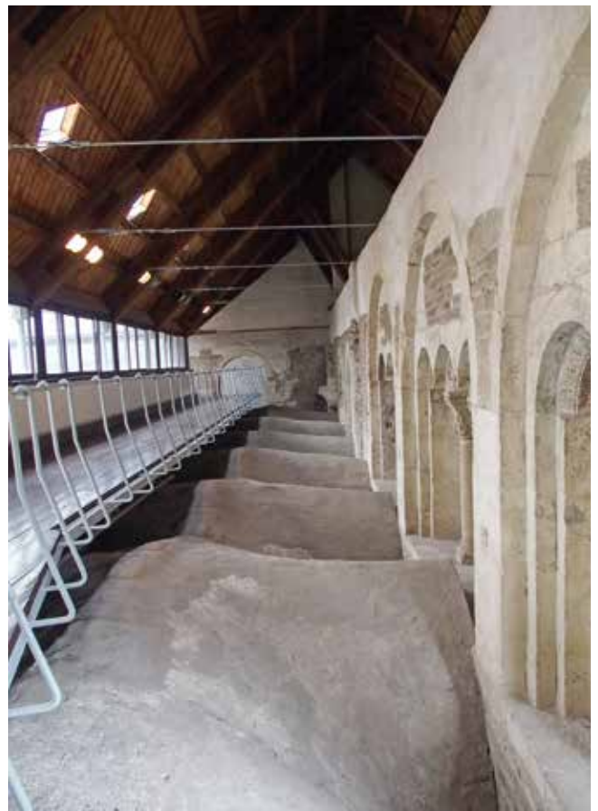
Figs. 4–6: Olomouc, Romanesque Zdik's Palace with roof and visitors' bridge from the 1980s, both intended to be replaced by glass-and-steel structures
