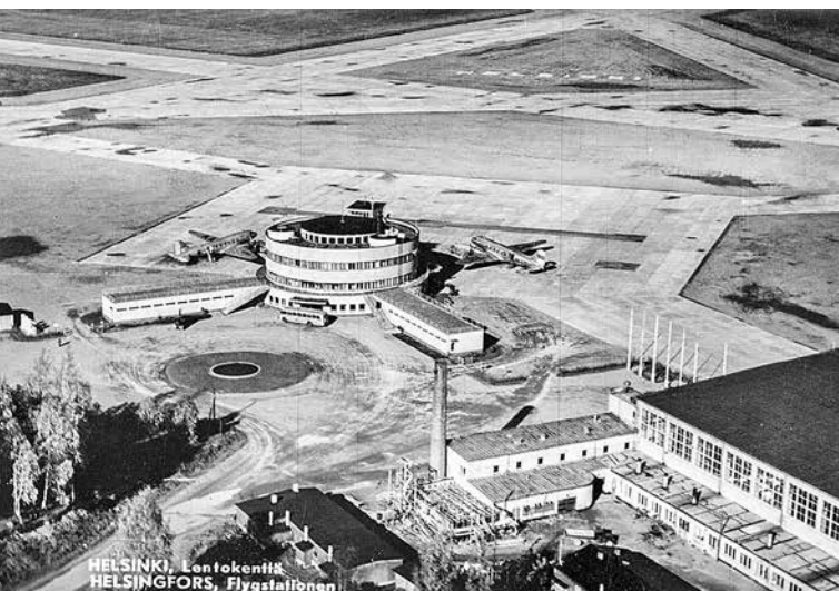
Fig. 1: Aerial view of Malmi Airport in 1948. In the centre is the circular terminal building with symmetrical wing buildings on the sides. In the foreground is the aeroplane hangar with its mono-pitched roof. (photo Veljekset Karhumäki 25.9.1948, Helsinki City Museum)
