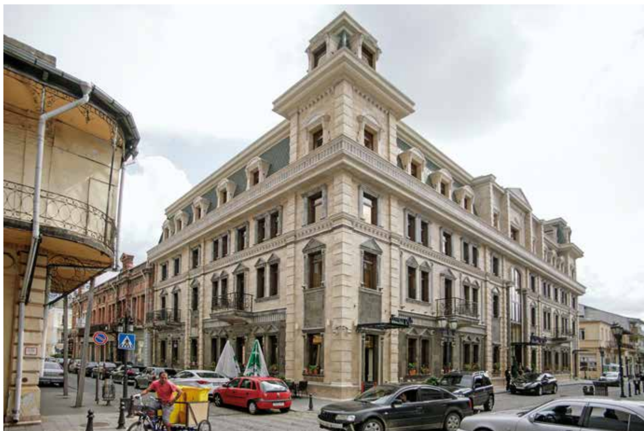
Fig. 6: Former Hotel London, imitating the reconstruction of a historic building (© Shota Gujabidze)
