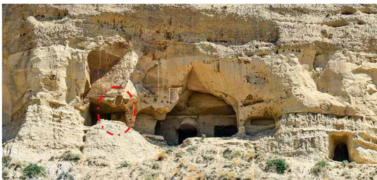
Fig. 3: Sabeerebi Monastery, slope façade with recent pillar collapse, situation in July 2019 (© Mikheil Elashvili)
