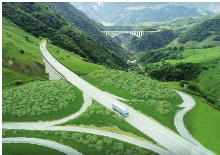
Fig. 6: Road plan: screenshot from the Road Department's own video of the proposed new road (© The National Trust of Georgia)
