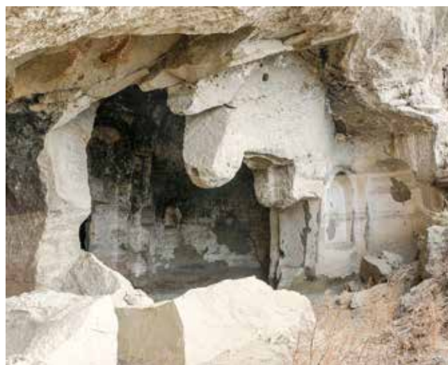
Fig. 4: Mravaltskaro Monastery, rock collapse (© Mikheil Elashvili)
