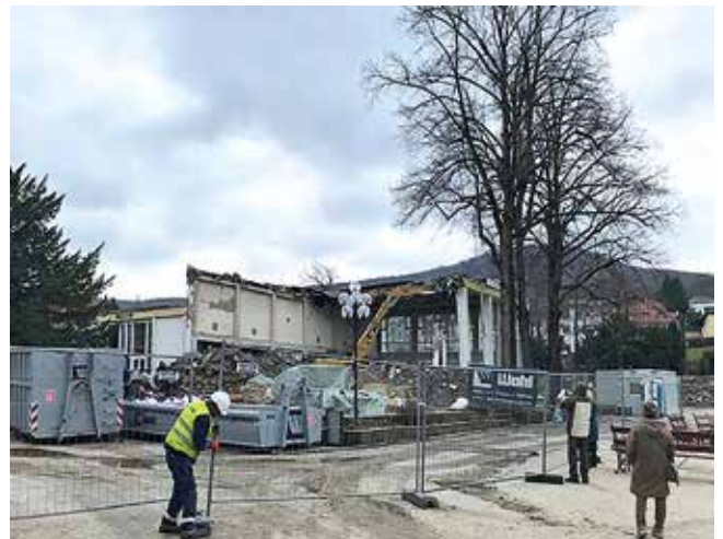
Fig. 3: Demolition of the spa buildings in spring 2020 (photo Michael Lentz)
