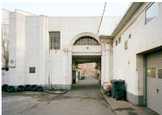
Fig. 2: Former west facade in the courtyard
