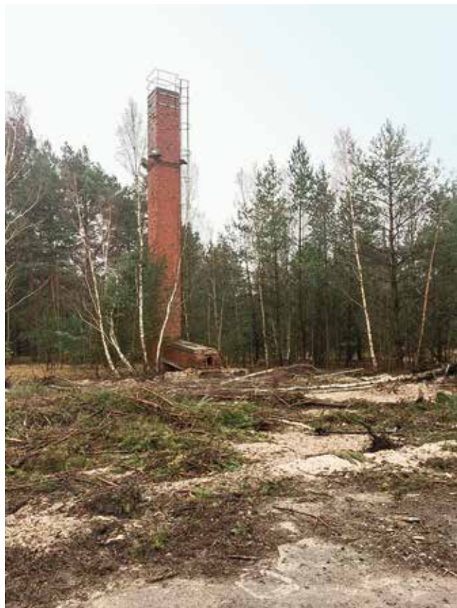
Fig. 2: Demolished building structure next to the IW (© P. Schneider/C. Röhl)
