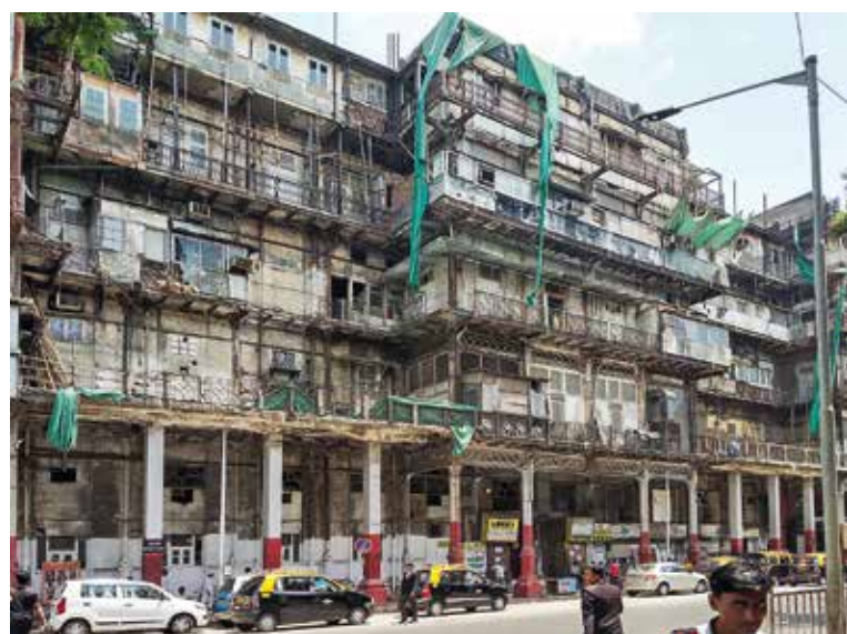
Fig. 6: Esplanade Mansion, main (north) facade, June 3, 2019
