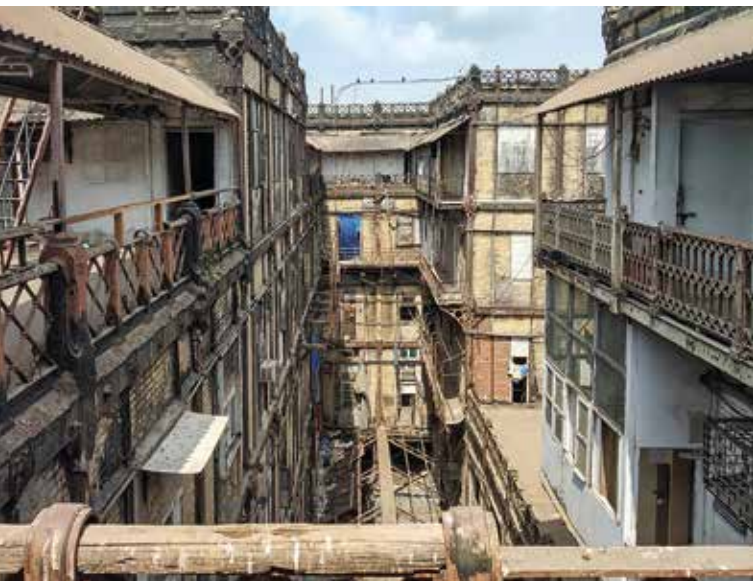
Fig. 7: Esplanade Mansion, internal courtyard, June 3, 2019
