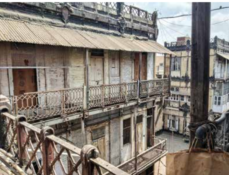
Fig. 9: Esplanade Mansion, internal façade details, June 3, 2019
