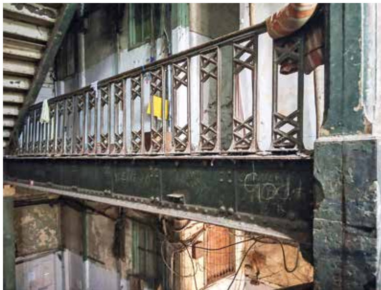
Fig. 8: Main staircase, wrought and cast-iron details, June 3, 2019
