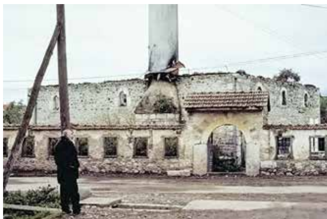
Fig. 1: Mosque in Deçan burnt during the 1998–99 War (© Riedlmayer, 2014)
