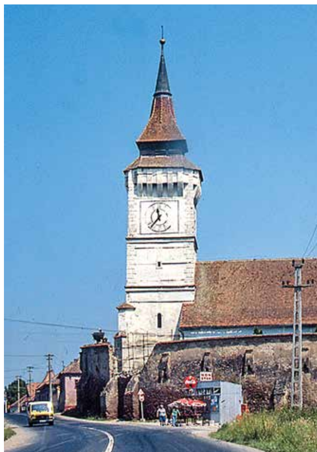
Fig. 3: The church in Rotbav before the collapse of the tower (photo C. Machat, 1998)
