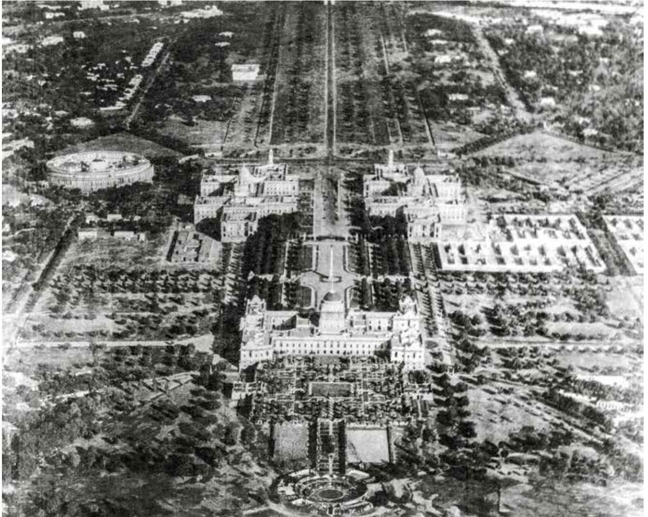
Fig. 3: Armature of the city identified as an important attribute that displays authenticity of form and material. This had remained unchanged over the years (© Department of Archives, Government of Delhi)
