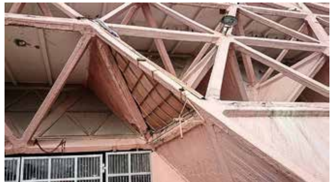
Fig. 6: External view of the lattice framework inspired by traditional jalis-sunbreakers and louvres (© Kiran Joshi, personal collection, September 2016)
