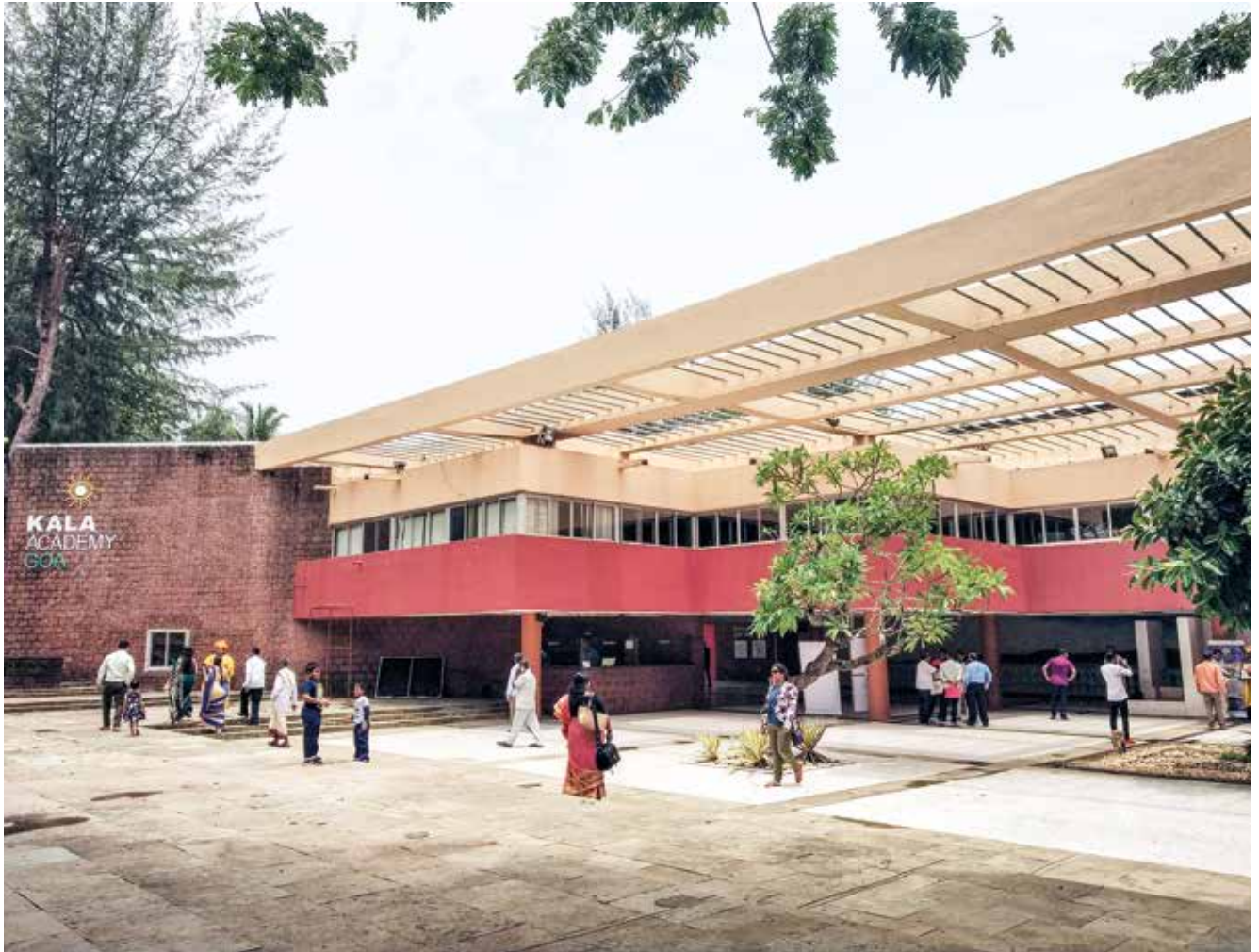
Fig. 1: The low-rise structure with a bamboo pergola extending across the entrance. The characteristic feature of this design is the open plan which seems to welcome everyone (© Sharad Apte, received through Charles Correa Foundation)
