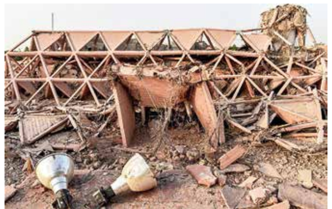
Fig. 9: Hall of Nations Demolished ( www.hindustantimes.com/photos-in-dia-newsthe-hall-of-nations-a-lost-heritage-of-delhi )
