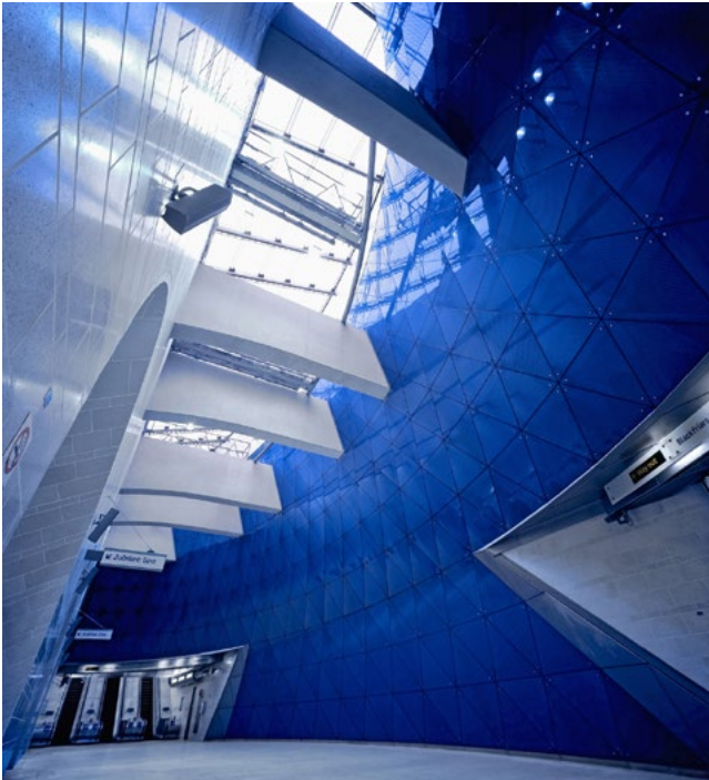
Fig. 3: Southwark underground station, close-up of curved blue glass screen designed by Beleschenko. The tiles are held by stainless steel 'spiders' connected to a steel frame
