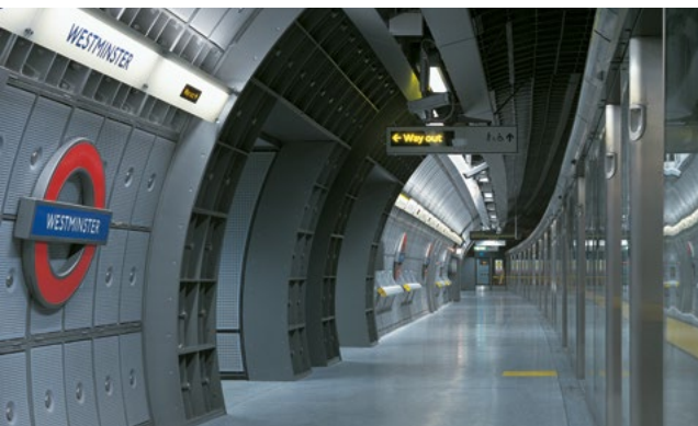
Figs. 5-6: Westminster underground station, 1999 by Hopkins Architects: A feat of mega engineering under Portcullis House next to the House of Commons, central London. Stacked banks of escalators hang from a dynamic network of flying concrete beams and steel tubes to create this vast dramatic backdrop.
