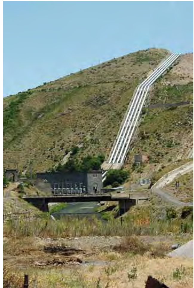
Fig. 6: Argel/Gjumush/Hydropower Plant (HPP), 1953 (architect: Tiran Marutyanyan)
