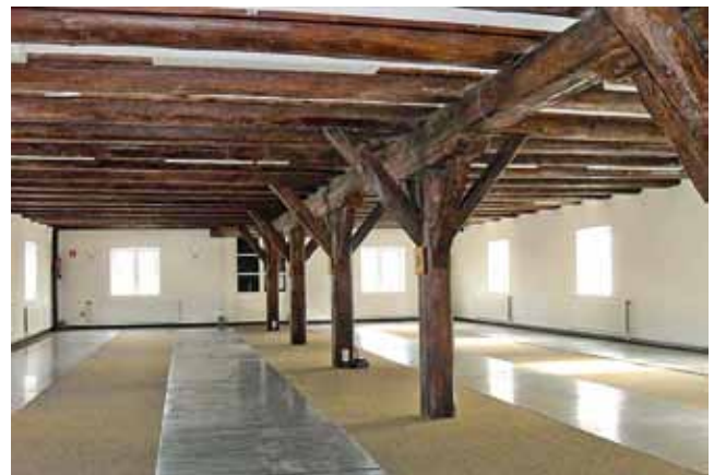
Abb. 5: Bremen, Vegesack, Thiele-Speicher um 1800, innen
