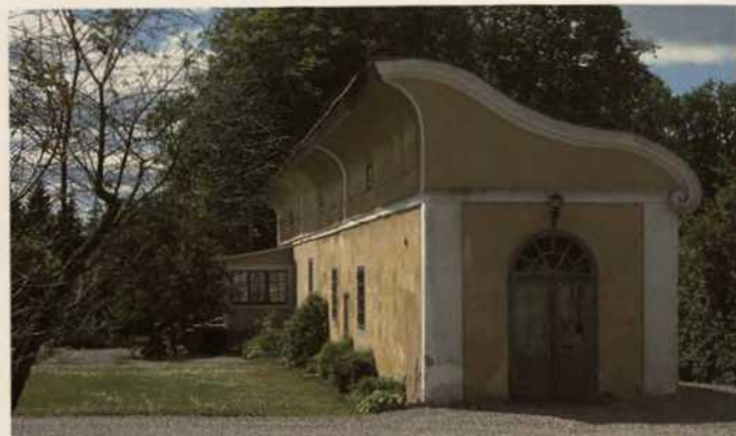
Fig. 18 Forcing house at Stora Wäsby, Stockholm, probably built in the late 18th century. Photo: Ingela Andersson, 2001
