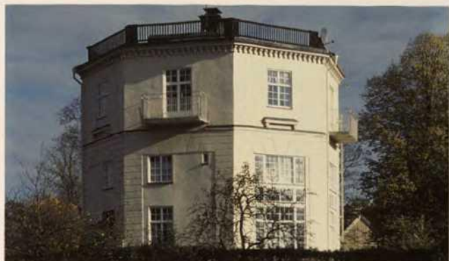
Fig. 8 Orangery at Stora Skuggan, Stockholm, used for palmtrees, built between 1796-99. Archibect: Jean Louis Desprez or Fredrik Magnus Piper. Photo: Ingela Andersson, 2001
