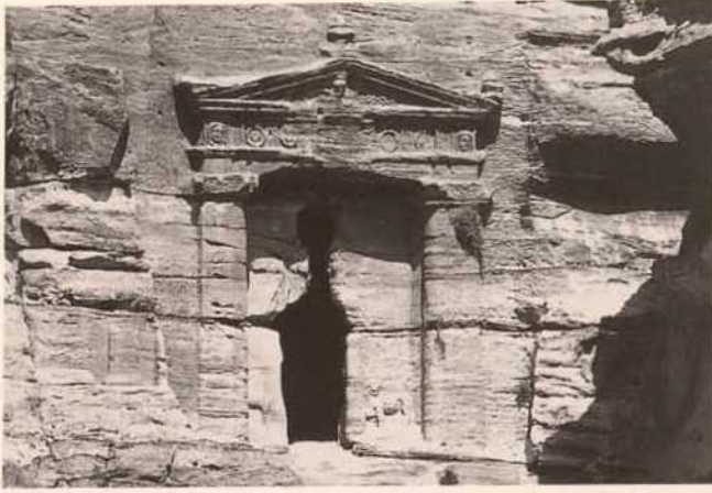
Abb. 4. Löwengrab, Riß an der Trennlage zweier Gesteinsschichten Fig. 4. Lions Tomb, crack following the line between two lithological layers
