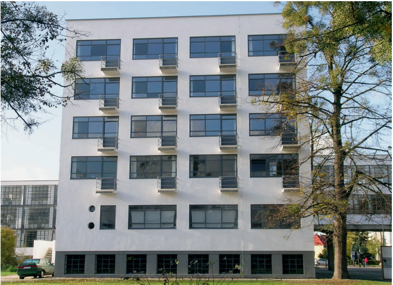
Fig. 2. Bauhaus atelier building after completion of restoration in 2006.
