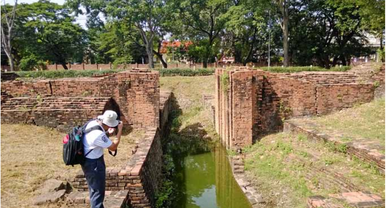
Fig. 3: Ayutthaya World Heritage site, where many canals have fallen into disuse, thereby restricting the water drainage capacity in the event of heavy rainfall
