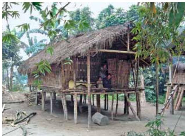
Fig. 4: Majuli Island, India: vernacular architecture built of bamboo on stilts, designed in response to floods that are regular phenomena in the region
