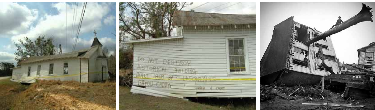
Fig. 4: Left and Centre: Historic church in Mississippi swept off foundations by Hurricane Katrina, right: A balloon frame wood house after the Johnstown Flood of 1889
