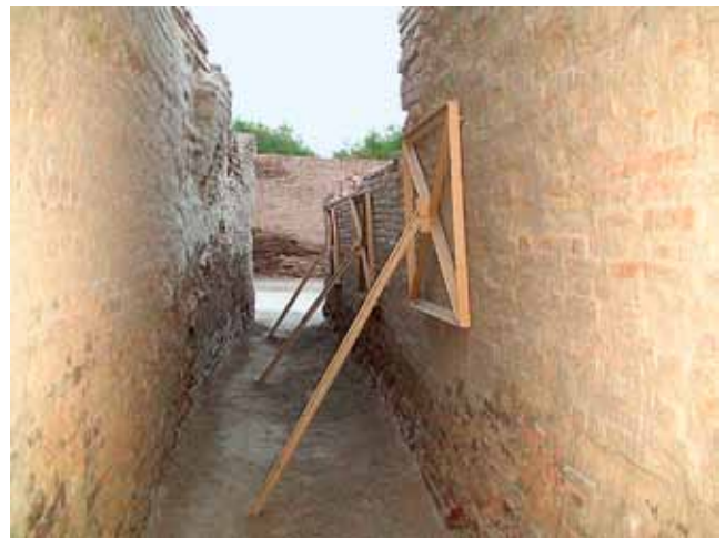
Fig. 17: Mohenjo-Daro, strengthening via shoring
