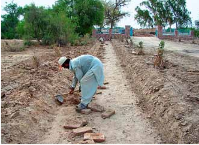
Fig. 13: Mohenjo-Daro, repairing of drains
