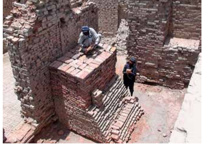
Fig. 16: Mohenjo-Daro, dry brick buttressing
