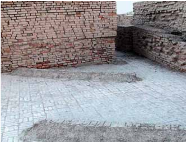
Fig. 14: Mohenjo-Daro, angular temporary barriers for preventing water flow
