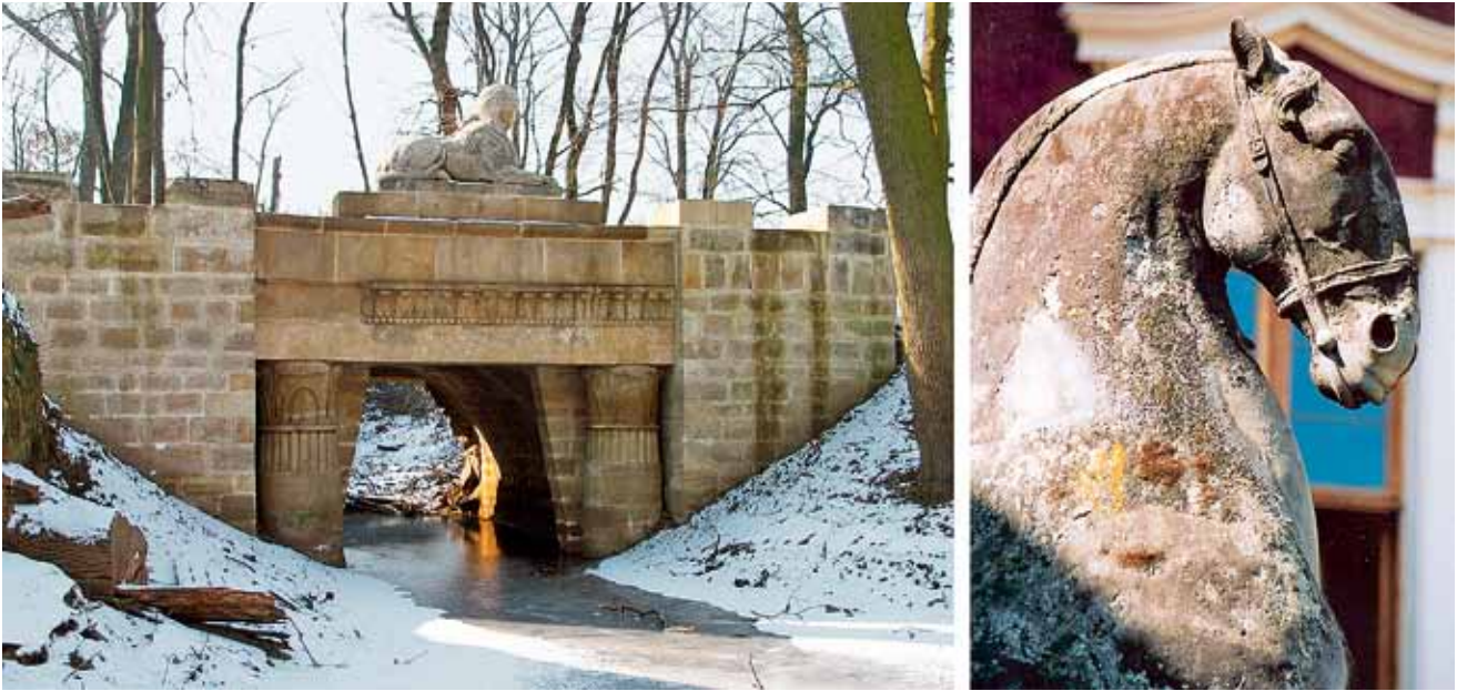
Fig. 3: Preventive restoration impact on the damage of monuments in the Château Veltrusy Park, near Prague: a) an appropriately restored bridge and sculpture, b) incorrectly restored sculpture
