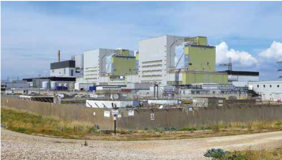
Fig. 6: Dungeness, Kent, to the right are the two Magnox reactors and to the left the later advanced gas cooled reactor (2016).
