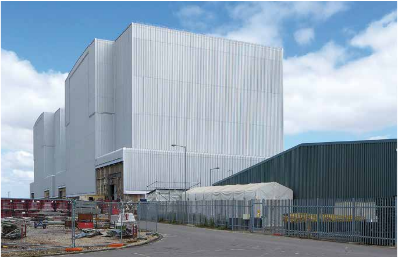
Fig. 10: Bradwell, Essex, after defueling the former reactor building has been reduced in height and reclad. It will probably remain in this form for a generation before final dismantling occurs (2017).
