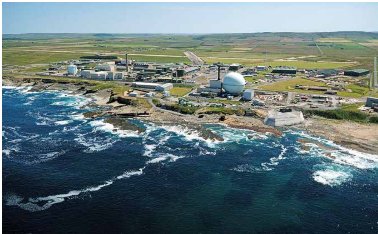
Fig. 1: View of Dounreay site mid 2000s.
