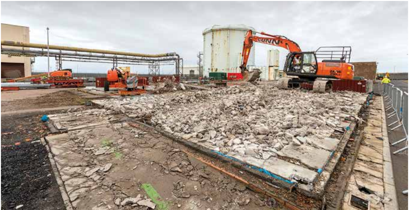
Fig 5: Decommissioning near DMTR.
