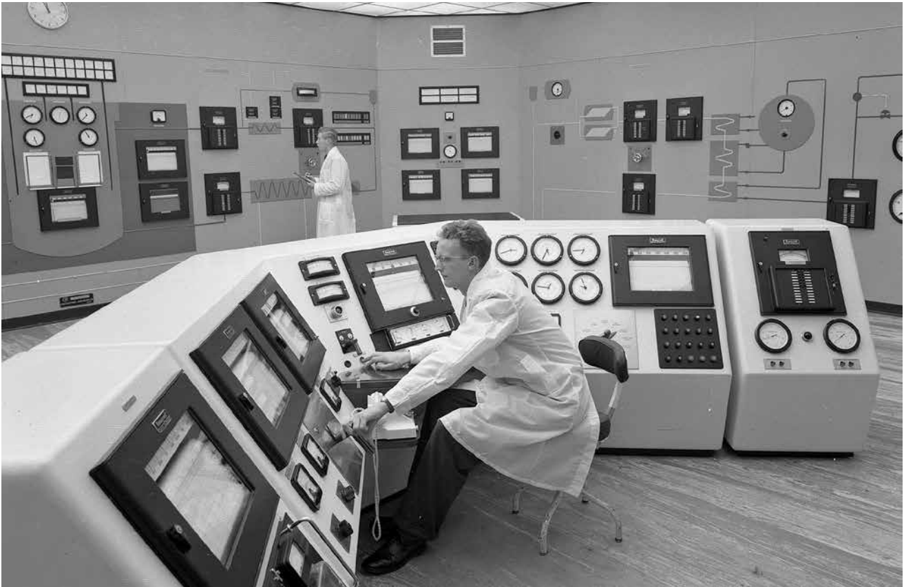
Fig. 3: DFR Control room, c. 1958.
