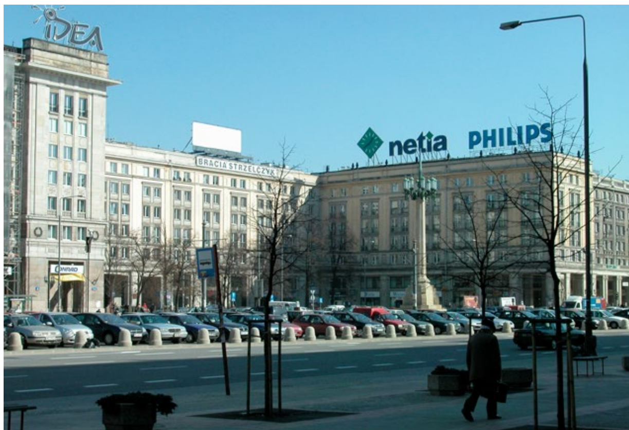
Fig. 2: Marszałkowska Residential District (MDM), Warsaw, south-eastern corner of Plac Konstytucji, Zygmunt Stepiański, Jan Knothe, Józef Sigalin and Stanisław Jankowski, 1949–1952
