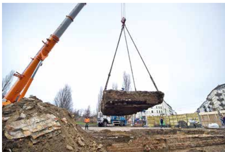
Fig. 10: Lifting of the vehicle lock, 2017 (© Torsten Dressler)
