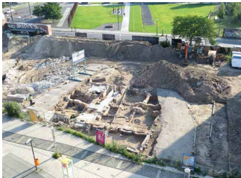
Fig. 8: Nordbahnhof excavation site, border installations east of Postenweg, 2017 (© Torsten Dressler)
