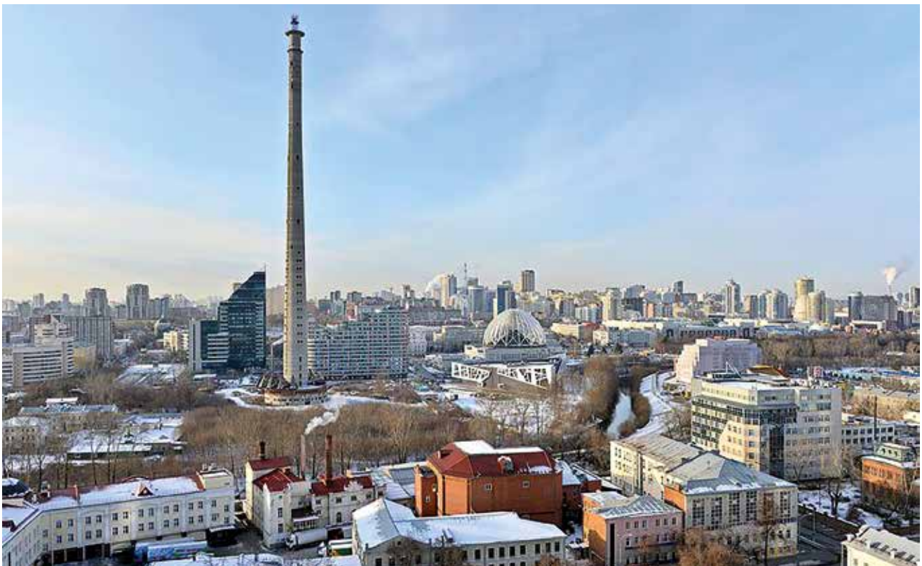
Fig. 1: TV tower in Ekaterinburg, demolished in 2018, general view
