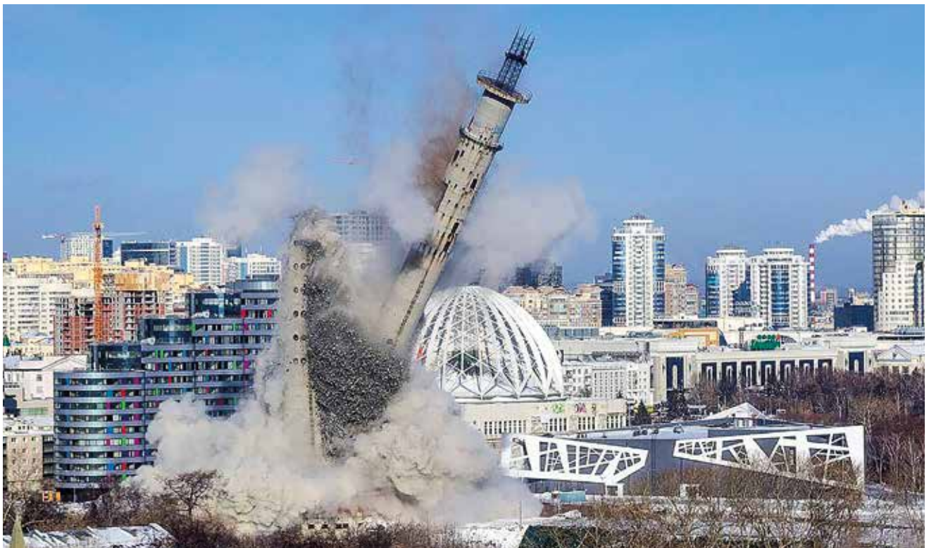
Fig. 4: The demolition ( http://www.brodyaga.com/pages/viewlarge.php?id=51040&cty=Ekaterinburg&place=Russia%20Sverdlovsk&region=Sverdlovsk )
