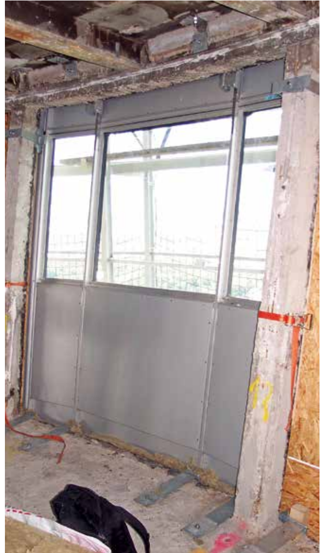
Fig. 10: Replacement of facade elements
