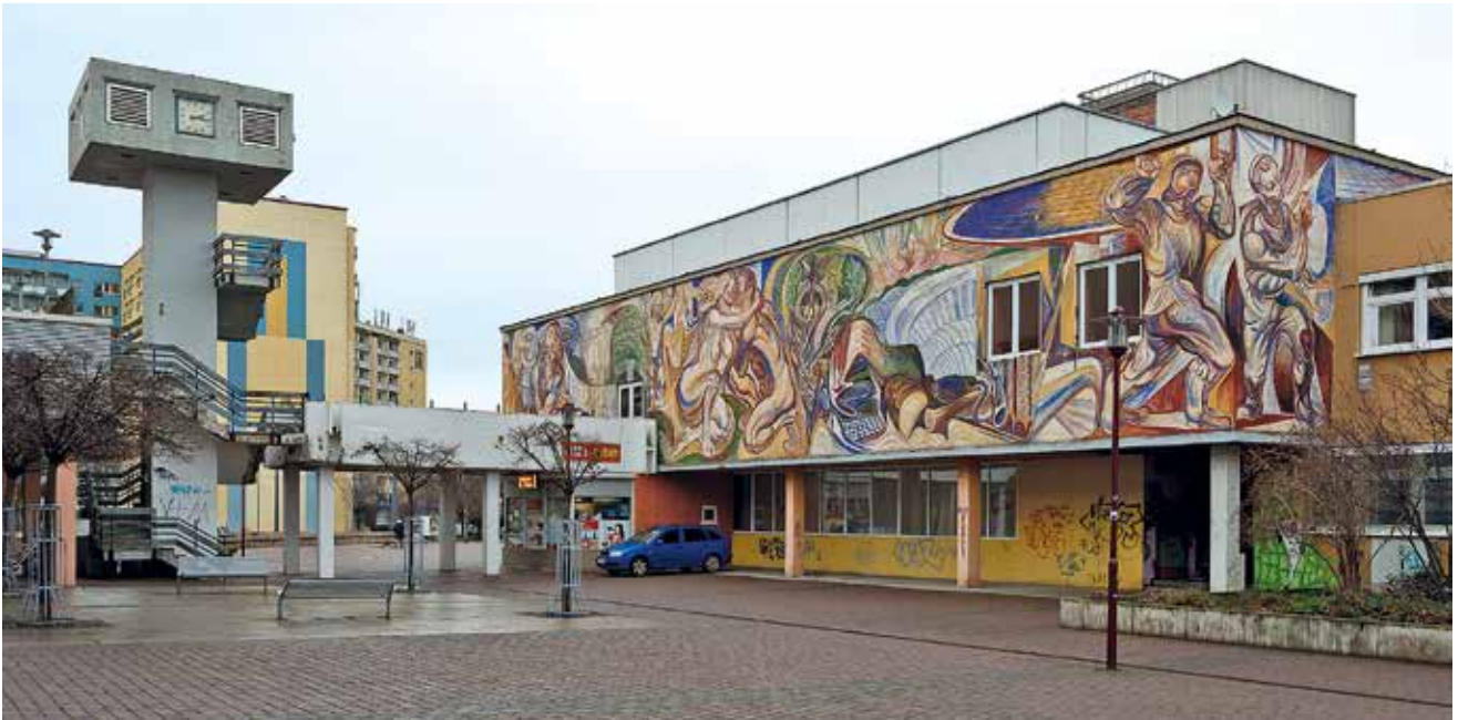
Fig. 7: Erfurt, residential area centre Rieth, former library building from 1973/74 with wall painting by Erich Enge. Condition 2014 Photograph: TLDA, Werner Streitberger, 2006
