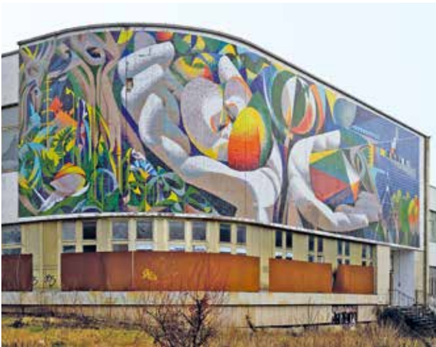
Fig. 6: Erfurt, Moskauer Platz 20, former cultural and leisure centre of the residential area Moskauer Platz from 1979–1983 with wall mosaic “Man, Nature and Technology” by Josep Renau; condition before demolition of the building in 2006 (photo TLDA, Werner Streitberger, 2006)
