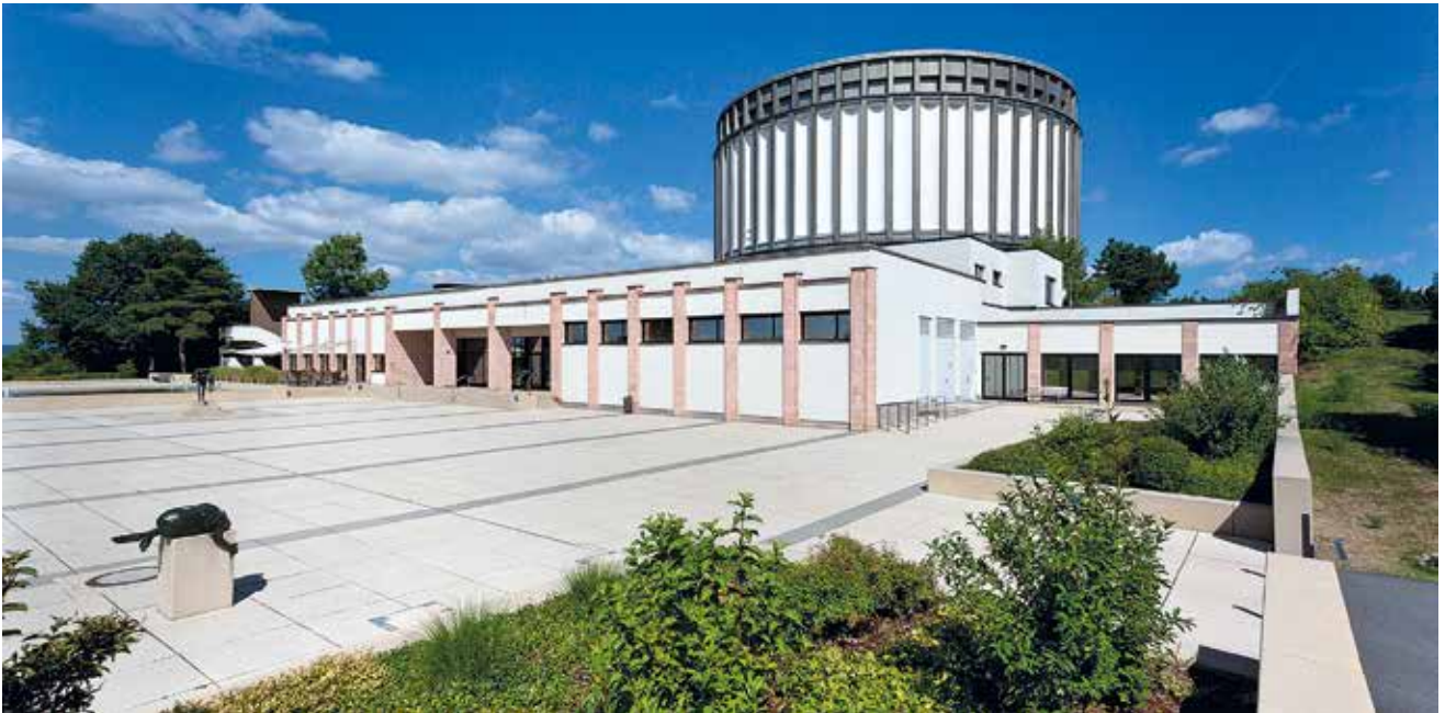
Fig. 8a: Bad Frankenhausen, panorama building on Schlachtenberg, 1975, condition 2013 (photo TLDA, Werner Streitberger, 2013)
