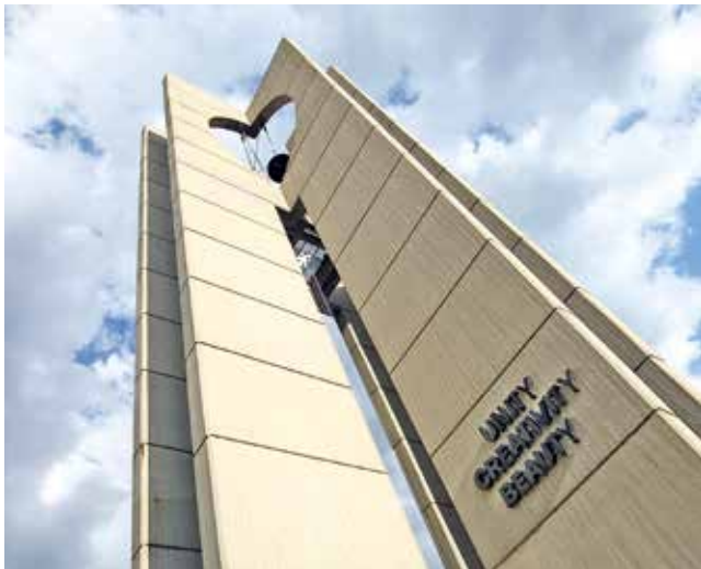
Fig. 6: The vertical body of the monument (Nikola Mihov for project ATRIUM)
