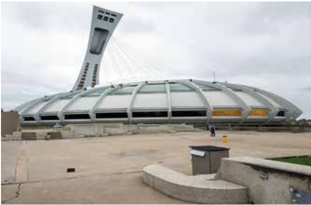
Fig. 6 The Olympic Stadium and its tower from the esplanade, currently being revitalized as a civic space and venue for events after decades of indifference
