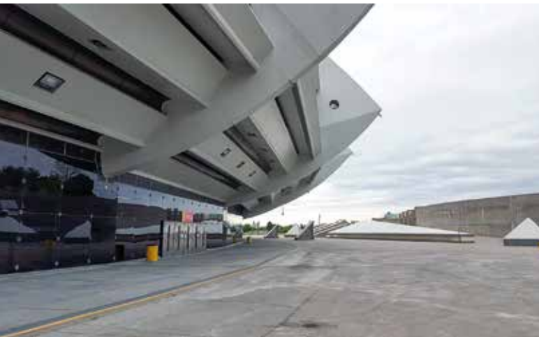
Fig. 3 The junction between the Stadium and esplanade showing the console structural system, its expressive use of concrete and original glass wall
