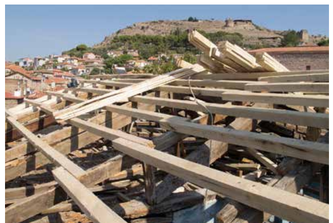
Fig. 6: Roofs are repaired in the most economic manner, saving as much of original elements as possible (Photo: DAI-Pergamon Excavation, Seçil Tezer Altay)
