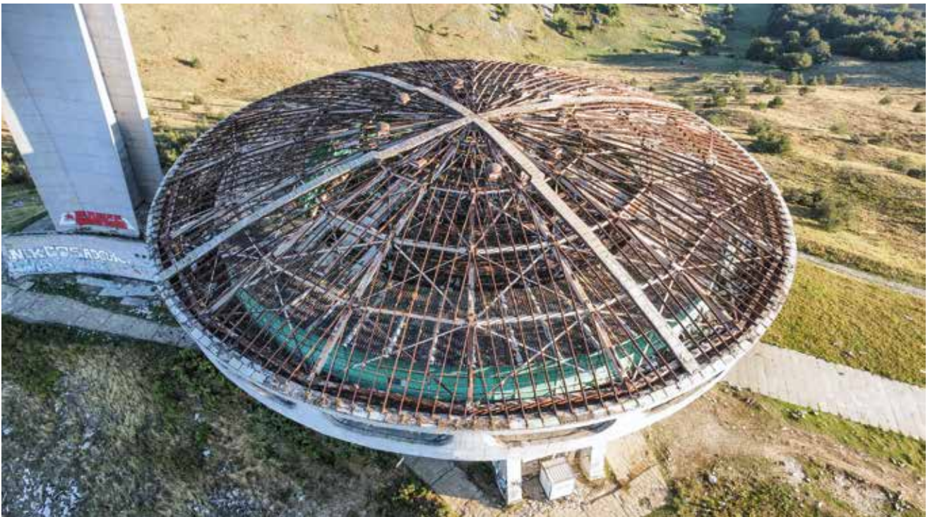
Fig. 15 Drone view of the cleared roof
